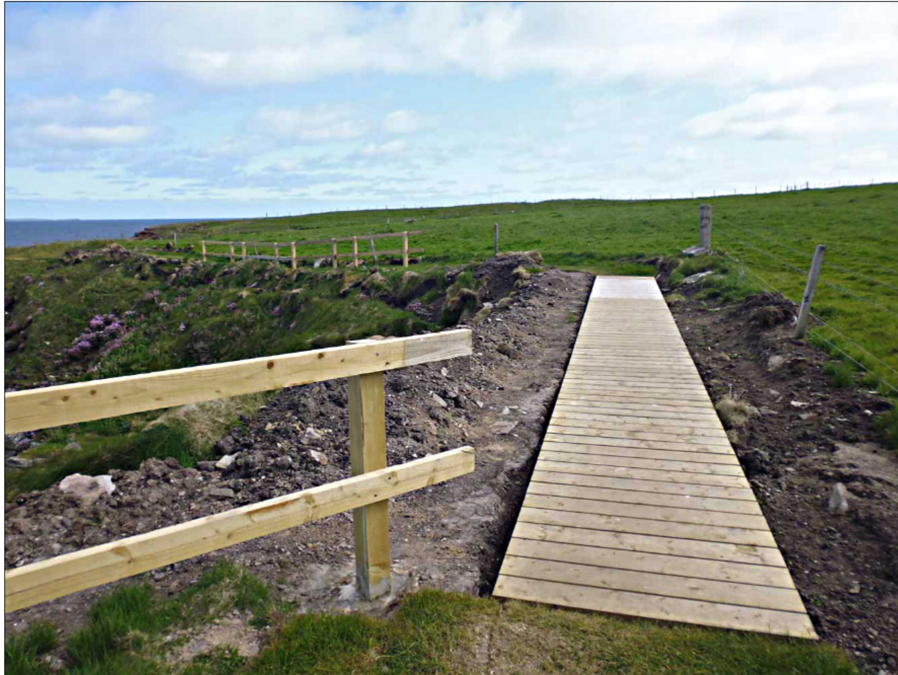
Staging has been laid where there were difficult or dangerous parts of the trail.
